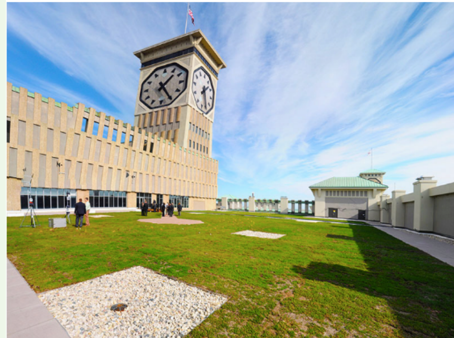
Rockwell Green Roof, Milwaukee (Credit: MMSD)
