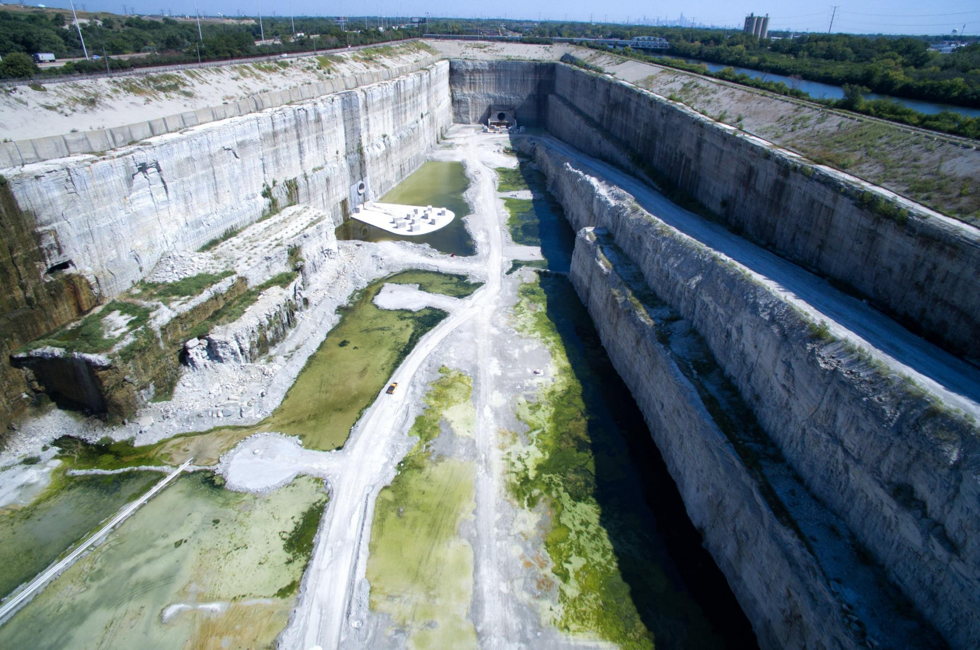
McCook Reservoir, Stage 1, 3.5 billion gallons
