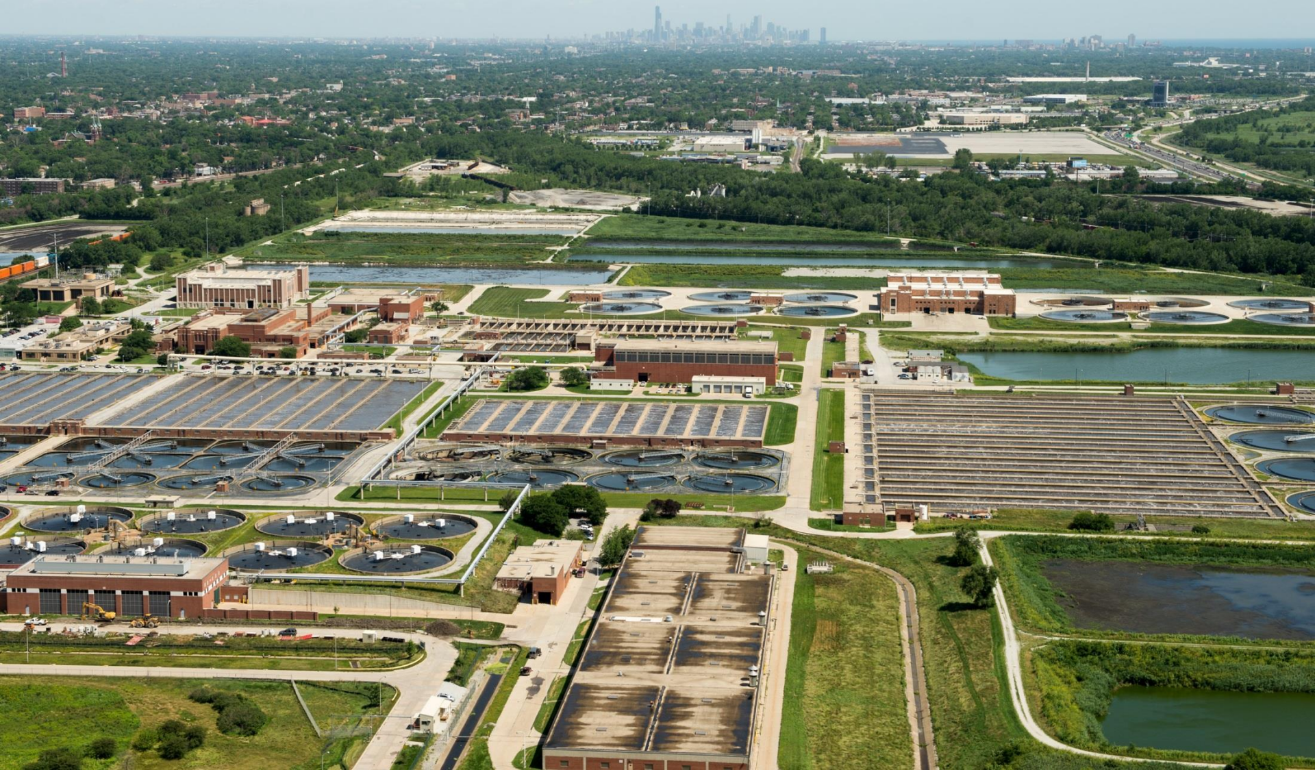
CALUMET WATER RECLAMATION PLANT
