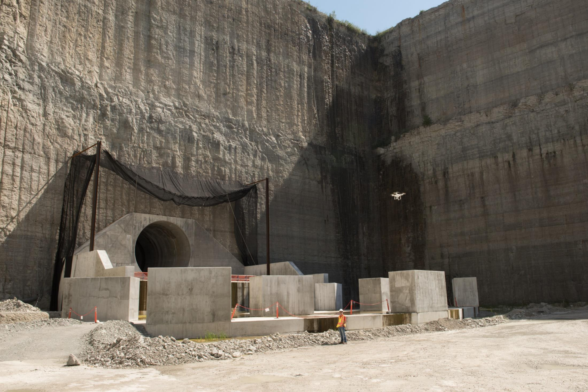
McCook Reservoir Mainstream Tunnel Portal
